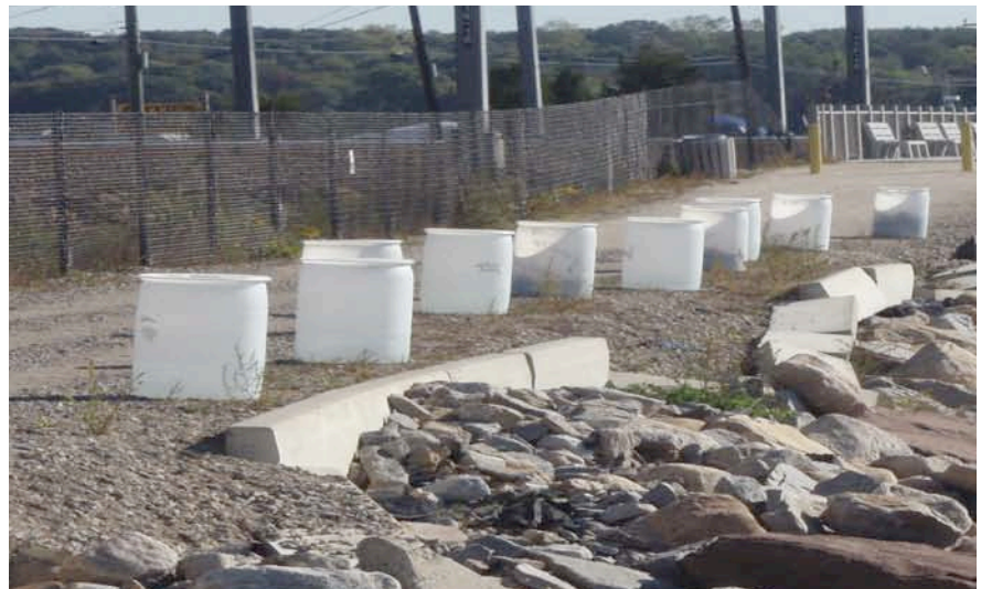
This collapsing section of Boardwalk in Niantic, shows both structures intended to provide stability and cement curbing originally intended to be decorative, but later undermined as rocks slumped and waves overtopped the walkway.
